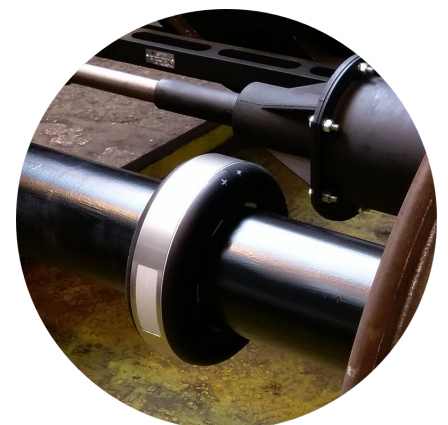
Photo from AxleRing installation
